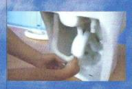
Install corrugated pipe. Elbow to S pipe fitting, straight section to kit assembly. Tighten hose clamp.
