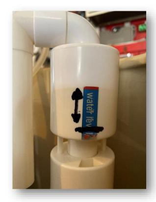
Toilet flush adjustments can be made by adjustment of set screws up or down. Apply teflon tape and secure lock nut. Correct adjustment of 1/16" - 1/8" from plunger. ( see photo )
