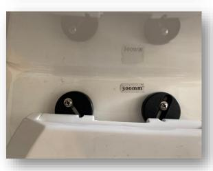
Remove seat by depressing both side buttons on quick release toilet.
