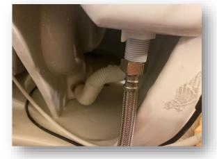
Remove toilet tank cover. Turn on water supply and let the toilet tank fill completely. Water level should be 1/4" - 1/2" from bottom of fan assembly.
