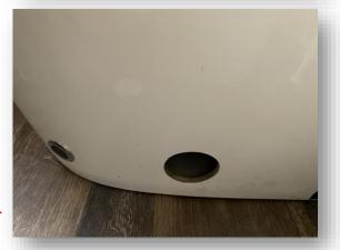
Use Side access holes to aid in toilet alignment on closest fitting studs. →
